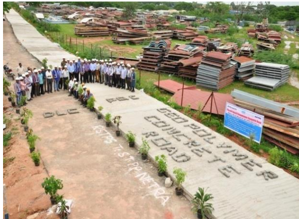
Fly Ash Geo polymer road construction at RSTPS
