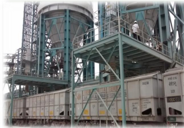
Dry Ash supply Rake Loading System
